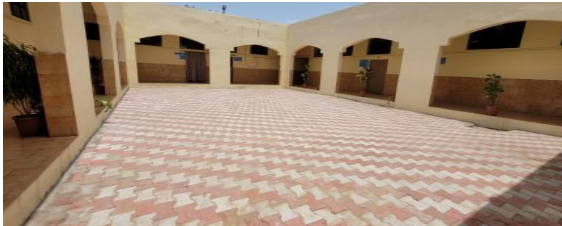
12000 Interlocking paver blocks placed in CPG-2 Building
